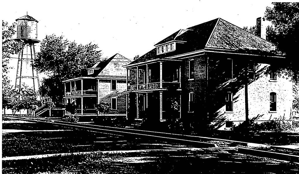
Employees' cottages. (NSHS-G335-7)
